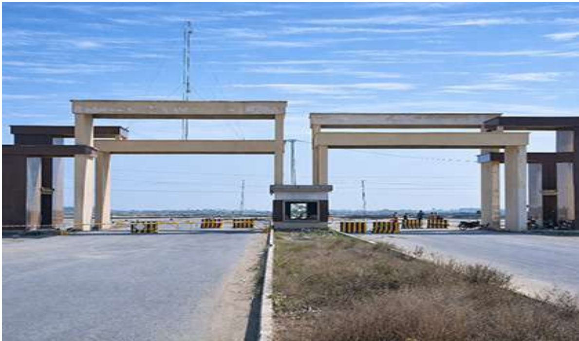
Figure 4 Allama Iqbal Industrial City, Faisalabad source: Faisalabad Industrial Estate Development and Management Company.
