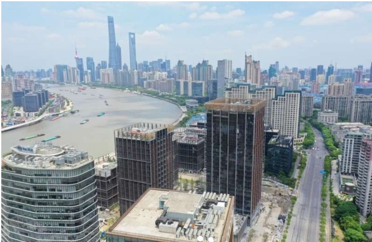
Figure 3 An aerial photo taken on May 22 shows the construction site of an office building project at the Binjiang Avenue in Pudong, Shanghai. The project represents the largest commercial building complex along Binjiang Avenue. Source:(People's Daily Online)
